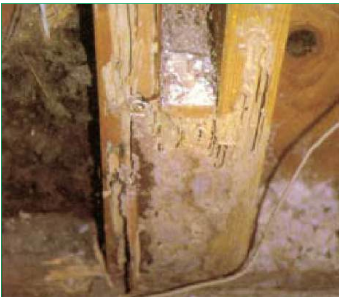
Figure 8. Formosan termite-produced carton nest in a structure.
