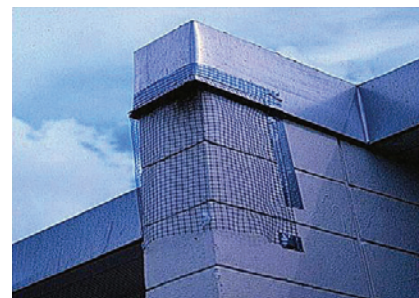
FIGURE 14 • Devices, such as bat netting, can be placed where birds or bats reside to allow one-way movement out of the cavity, thus they can also be used for exclusion.
