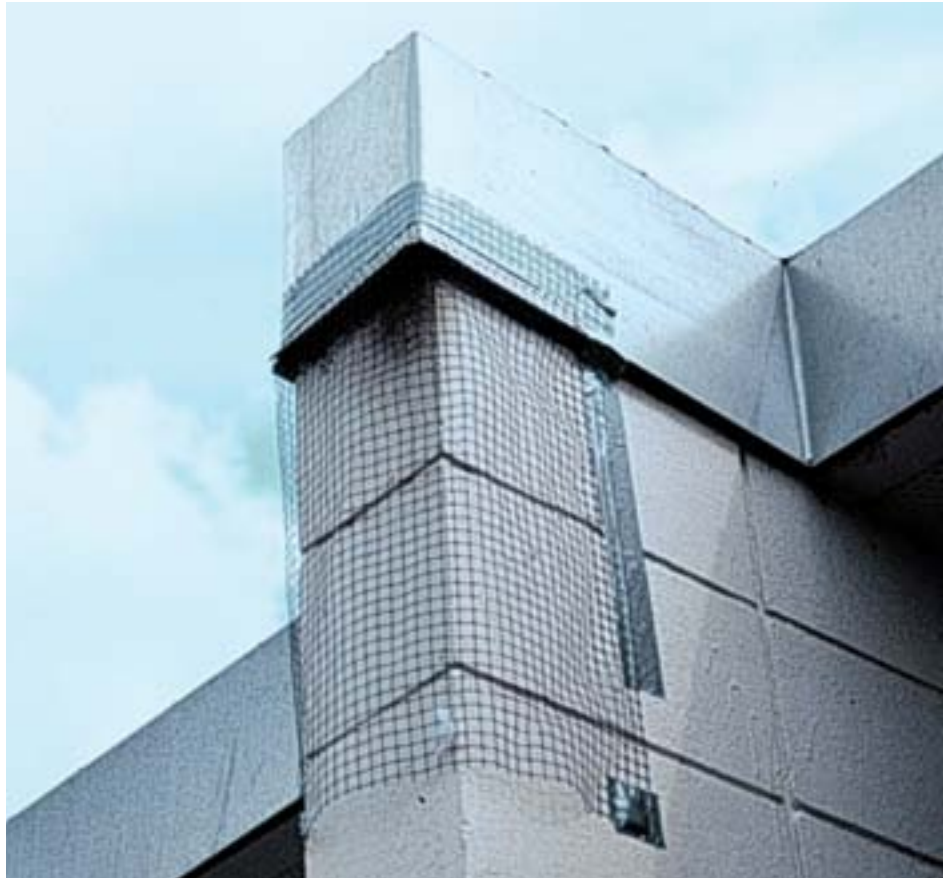
Figure 14. Devices, such as bat netting, can be placed where birds or bats reside to allow one-way movement out of the cavity, thus they can also be used for exclusion.
