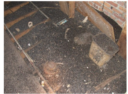
Guano needs to be cleaned up by a professional in bio-remediation. Remember safety first.
