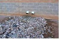
Incorrect placement of splash-guards (left) leads to puddling of water near building foundation and soil erosion — Shaku Nair, University of Arizona
